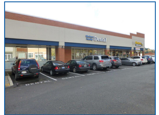
West view of Center
